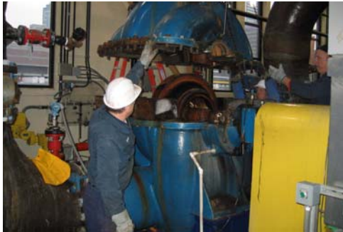
650 HP Horizontal Split Case Pumps being taken apart for rebuild
